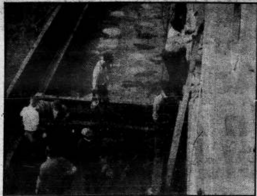
Workers clamber in and out of railroad cars to get to the Steel Navigator's ladder at the Pennsylvania RR docks in Baltimore.
