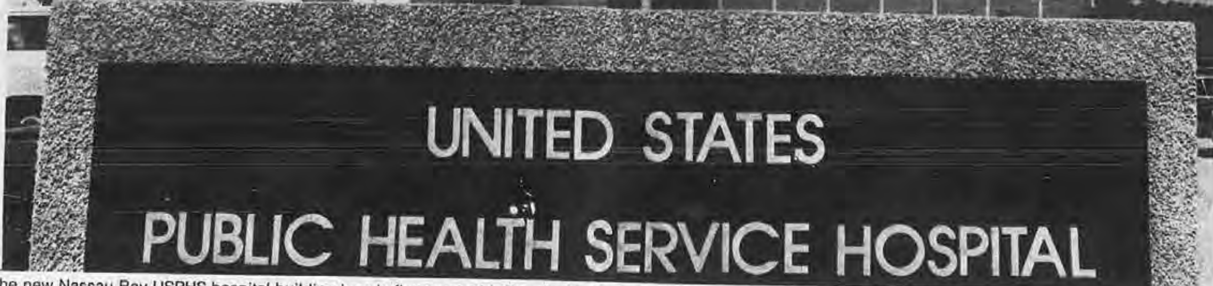
The new Nassau Bay USPHS hospital building is only five years old. Shortly after it was built, it was no longer needed for its original purpose as a community hospital. Its opening this month as a replacement for the deteriorated Galveston facility has preserved much needed services for American seamen and other PHS beneficiaries in the Texas coast area.
