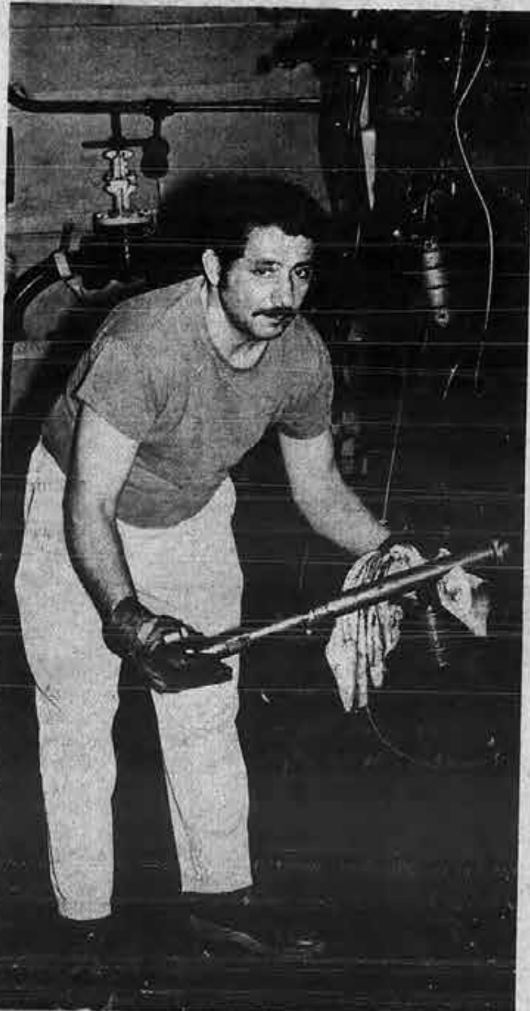
Fireman-Oiler-Watertender Mohamed Omar changes burners in the boiler.
