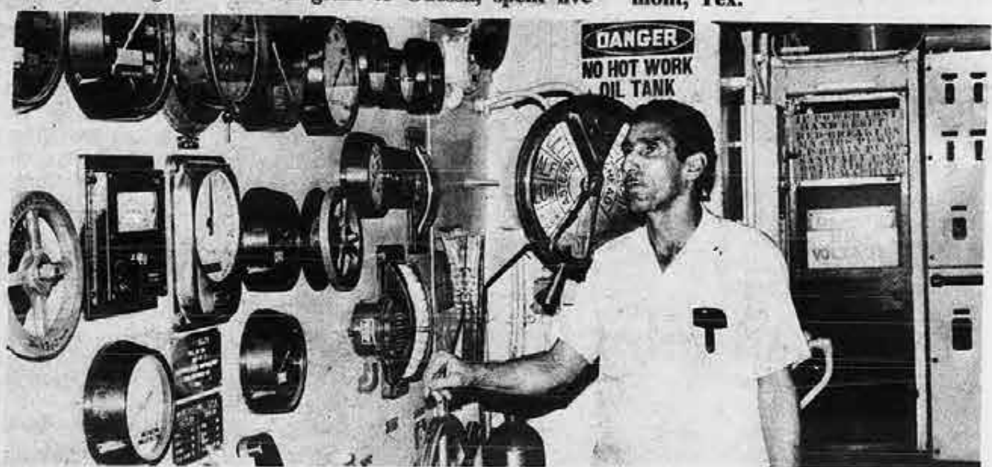
Oiler Oscar Ortiz checks gauges in engine room to make sure everything is running properly aboard the Achilles.
