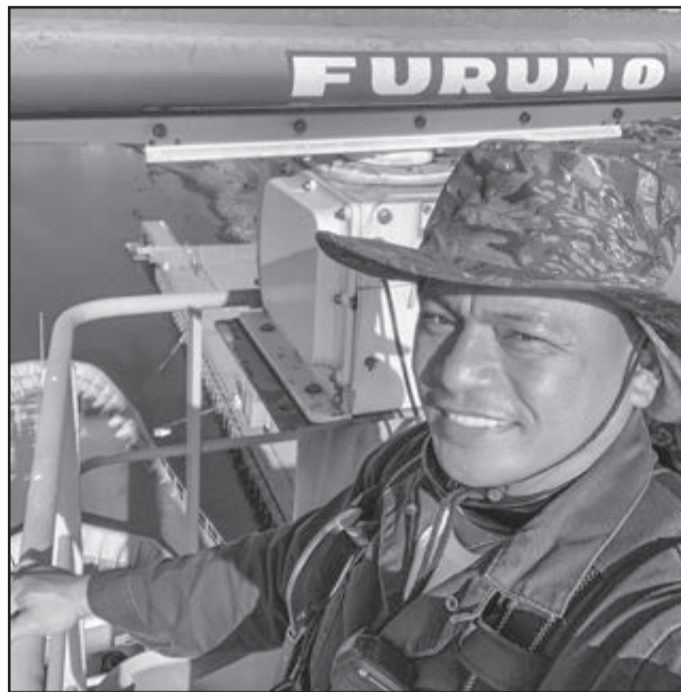
Recertified Bosun Ritche Acuman performs preventive maintenance for radar foundation aboard the USNS Algol (Ocean Duchess) in San Francisco.
