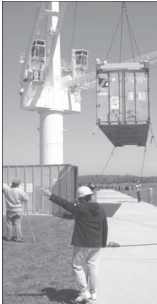
Cargo Handling and Crane Operations — Included in the third week of the government vessels course of study, this class provides students with a comprehensive examination of cargo handling situations aboard vessels. The operation and maintenance of equipment is stressed, along with safety precautions and requirements. Students are given opportunities for practical application.
