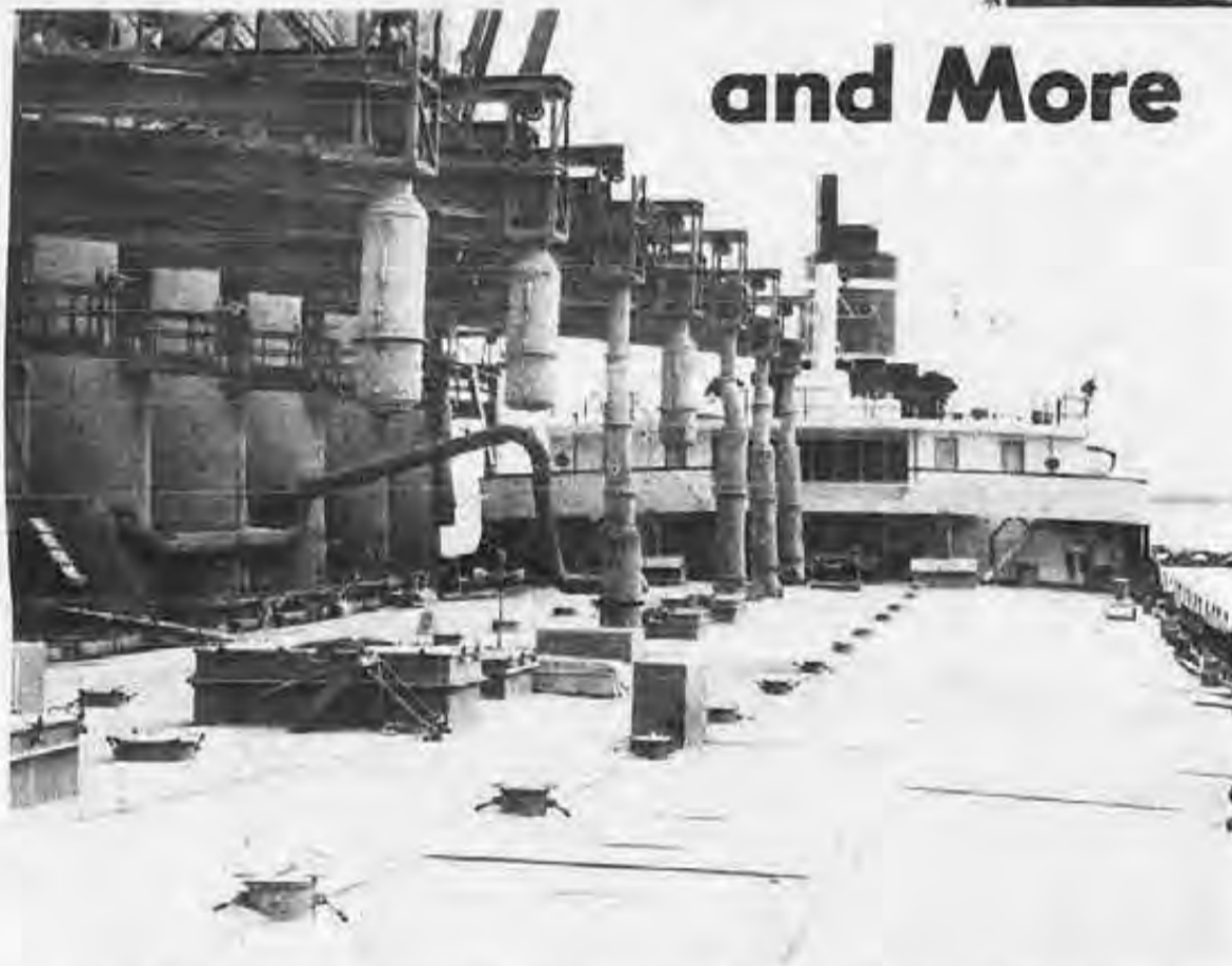
A view of the loading pumps on the J.A.W. Iglehart . The 16" wide hoses, four of which are in use here, are hooked-up to on-shore silos in different ports to unload the cement.
