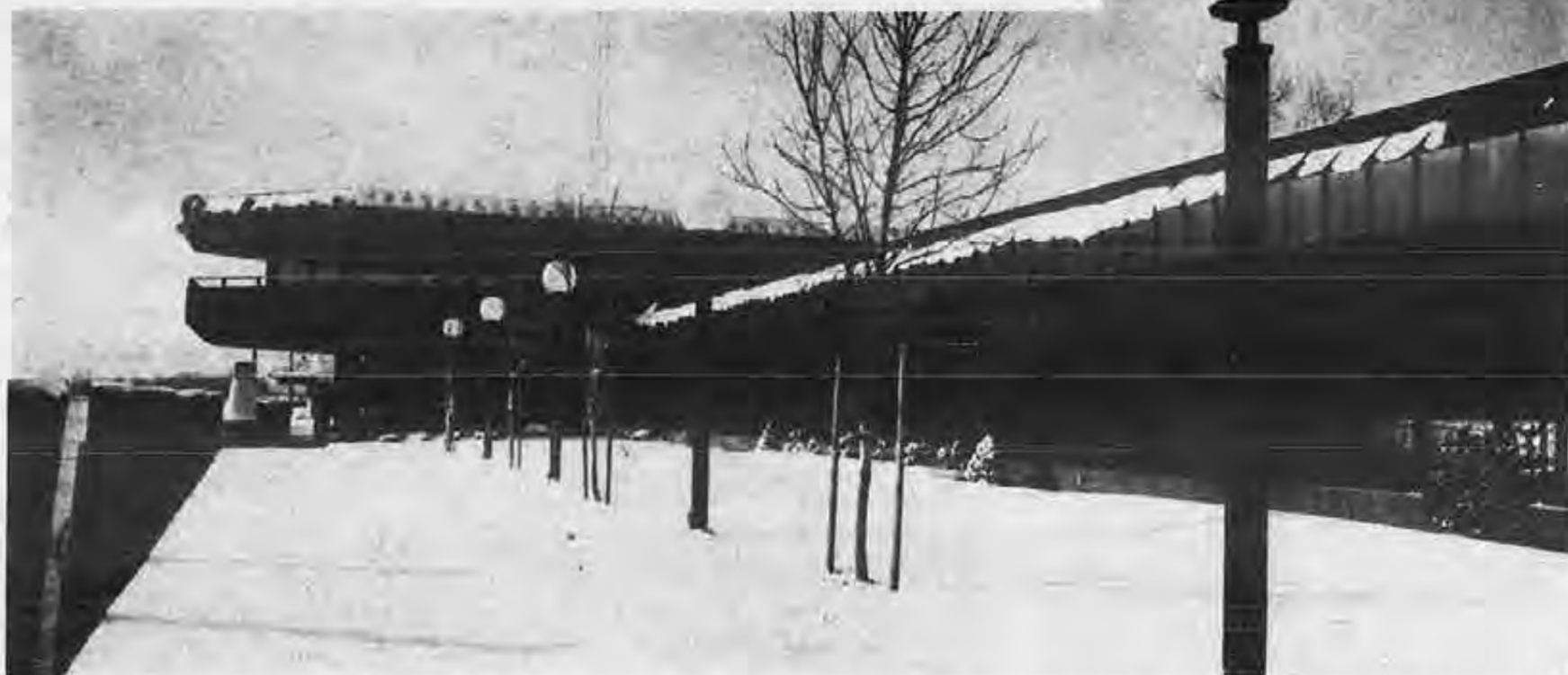
The new hall in Algonac, Mich. officially opened on Jan. 3. This hall is built right on the St. Clair River, which can be glimpsed through the wood pilings that front the building. The large room on the hall's second level holds a kitchen and conference area and is built atop the hall's boathouse.
