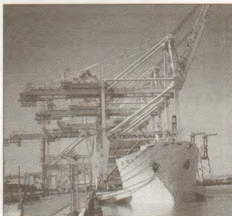
These giant cranes are a recent addition to the port of Oakland and are designed to accommodate the newest generation of container ships. They can each lift 65 long tons at one time and can reach 201 feet over a ship, hoisting at a speed of 230 feet per minute and with a capacity to load more than 30 cargo containers in an hour.
