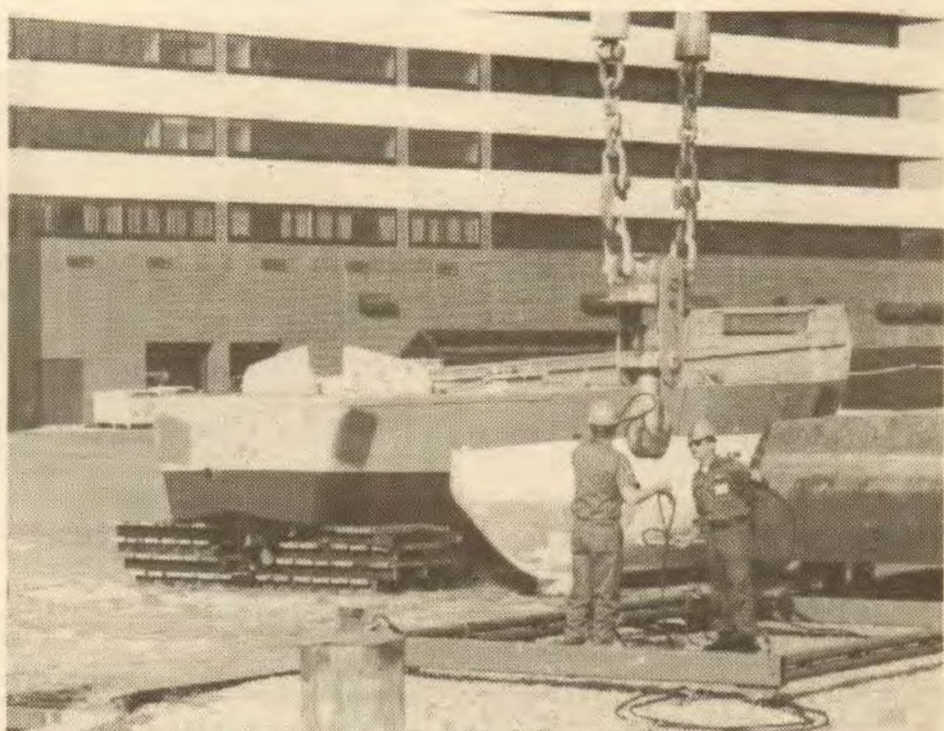
Melvin Hewitt (l.) and Gerald LeBar preparing to hook up the spreader in twin operation.
