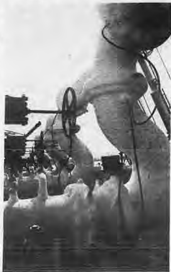
Just a short distance from Bontang is the loading site for the LNGs. Note the ice on the lines as the 287 degree below zero liquefied gas is loaded into the LNG Gemini's tanks.
