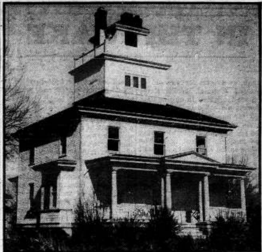
The Liston Range Front Light is an example of one of the older and simpler lighthouses in the US. This one, located at Middletown, Delaware, is simply an old house, with the blinker light installed in the tower. It has a fixed blinker instead of a sweeping light, thus making this type of installation practical. The keeper and his family have their quarters in the lower part of the house. This type of installation is fairly easy on the keeper and his family because of the size of the building.
