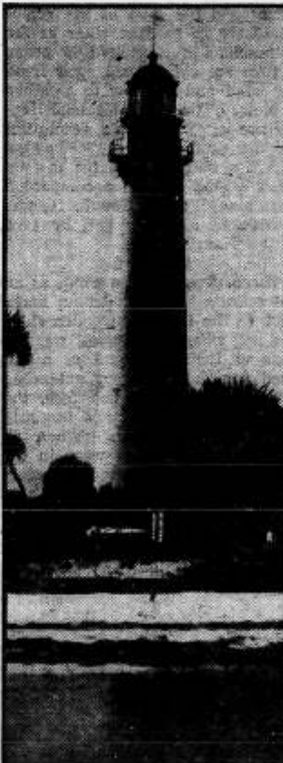
The Egmont Key Lighthouse, on a tiny sandy island, is a familiar sight to those entering the ports of Tampa and St. Petersburg, Fla. The first light was erected on this island in 1848. The present tower was put up in 1858, and is still in operation after almost 100 years of constant service.
