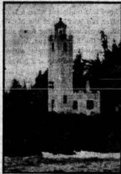
The "Honeymoon Castle," the Tree Point Light Station off the Alaskan Coast is hard to beat as far as a lonely location is concerned. Now manned by a Coast Guard Chief Boatswain's Mate and his former SPAR bride, the installation is six hours' sailing from the nearest small town. It is located on a barren peninsula-island and just about cut off from civilization.
