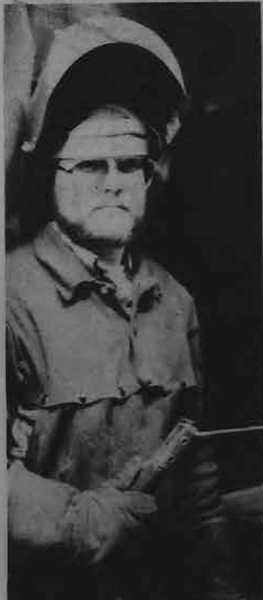
Jimmy Skubna's electric arc welds a four inch pipe.
