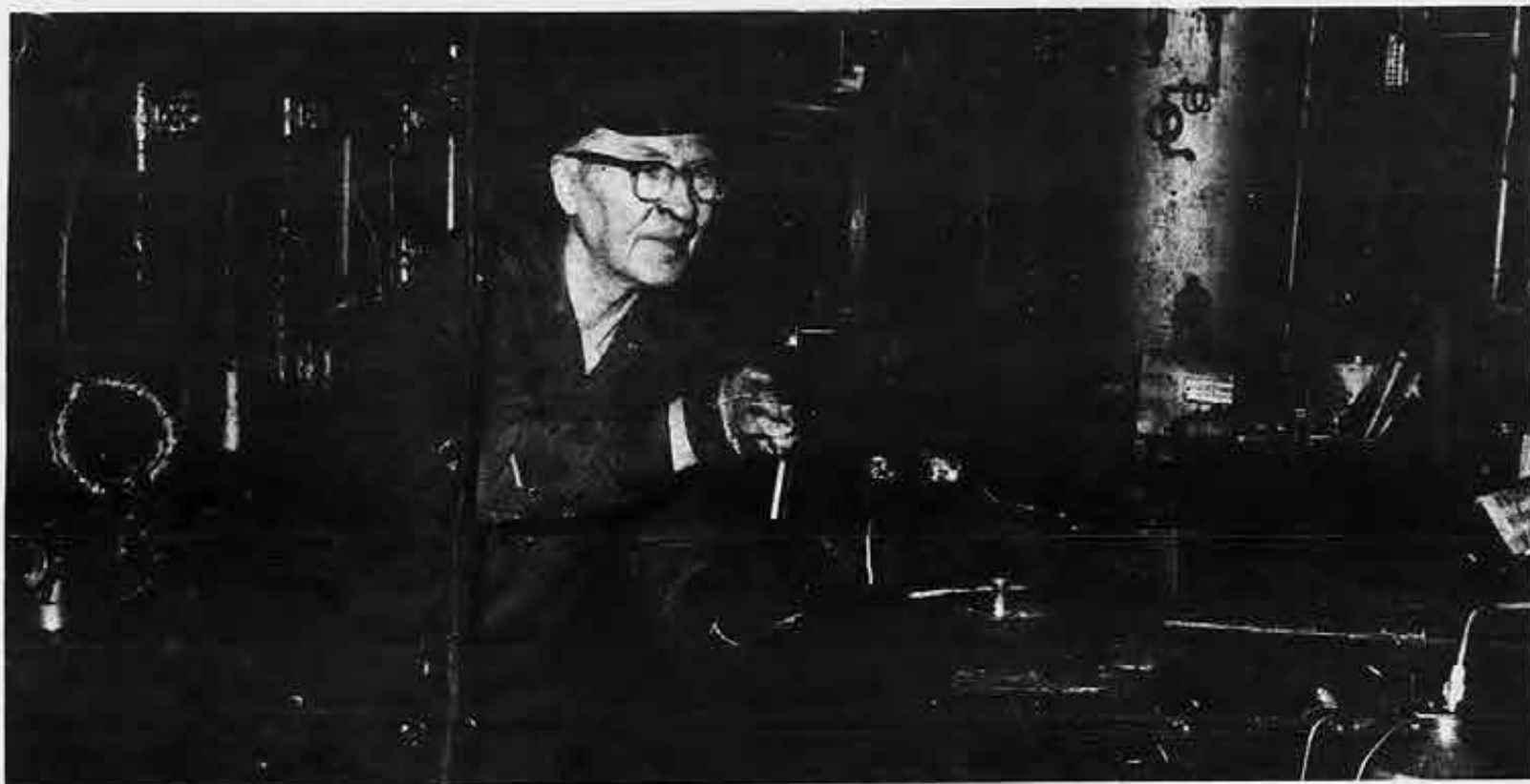
Seafarer Francis Buttas stamps out flange on damper that was stripped and needed a new thread. Buttas sails as fireman aboard the John T. Hutchinson .
