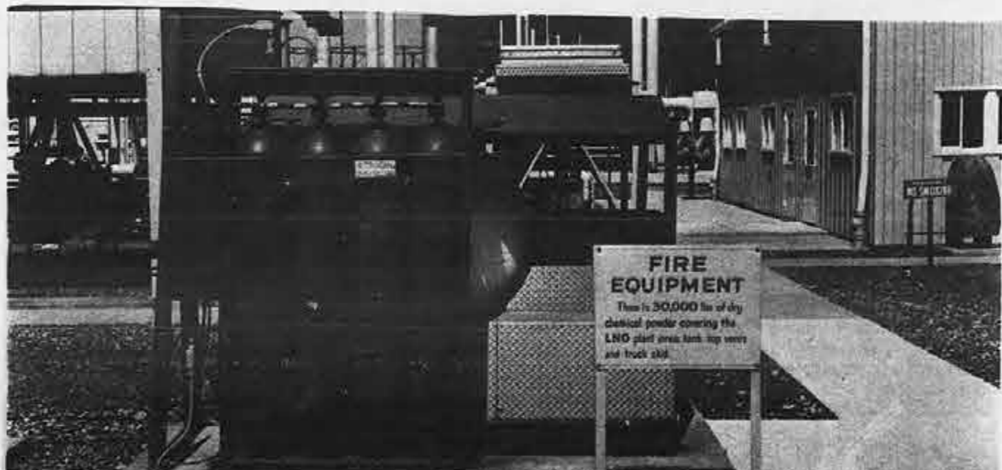
During the Lundeberg School's LNG Program the men take a field trip to a "peak shaving" LNG plant in Baltimore. To the left is a pre-treatment system which prepares natural gas for the supercooling process needed to convert it to its liquid form. Above is (bottom) an automatic chemical firefighting system which will help protect the plant in the event of a gas fire and (top) the central station which monitors and controls the entire plant.
