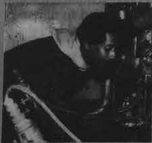
DEU Eladio Cruz checks steam and oil valves. A ship's delegate, the New Yorker has been sailing for 14 years.
