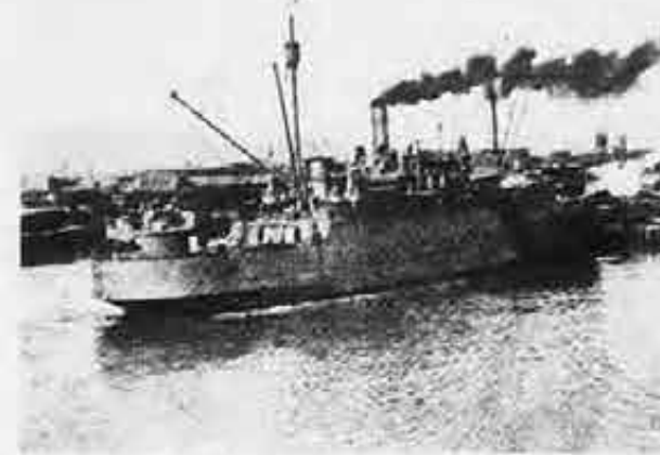
A Hough-class ship underway and headed for the shipyard for repairs. Green timber, inexperienced shipbuilders, overpowered plants all contributed to the problems of the ships. The 3,500-ton cargo capacity of these coal-burning ships was drastically reduced by the enormous amount of bunkers they had to carry.
