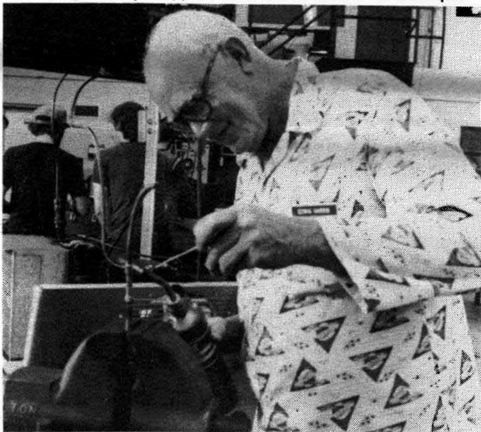
Edwin Harris uses a propane torch to solder a soft copper refrigeration tubing swaged joint.
