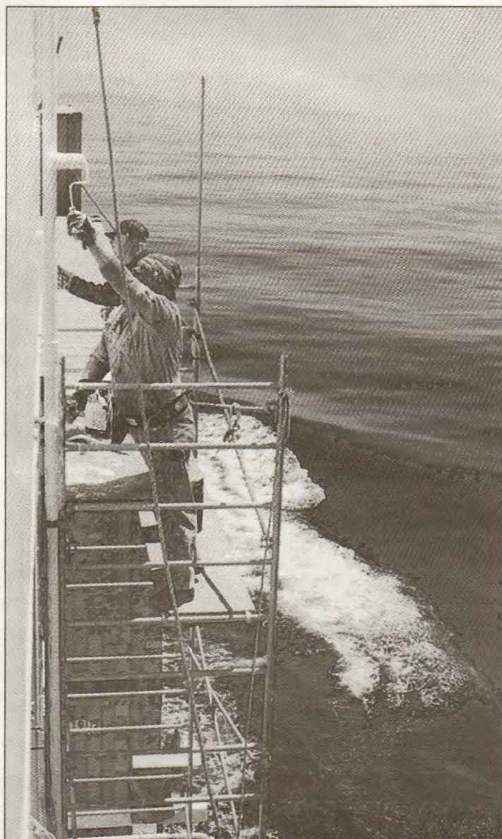
ABs Tony Carvalho and Rod Clark paint the side of the house on the CSX Anchorage , off the coast of Canada. The photo was sent to the Seafarers LOG by Chief Engineer Bruce Sherman.
