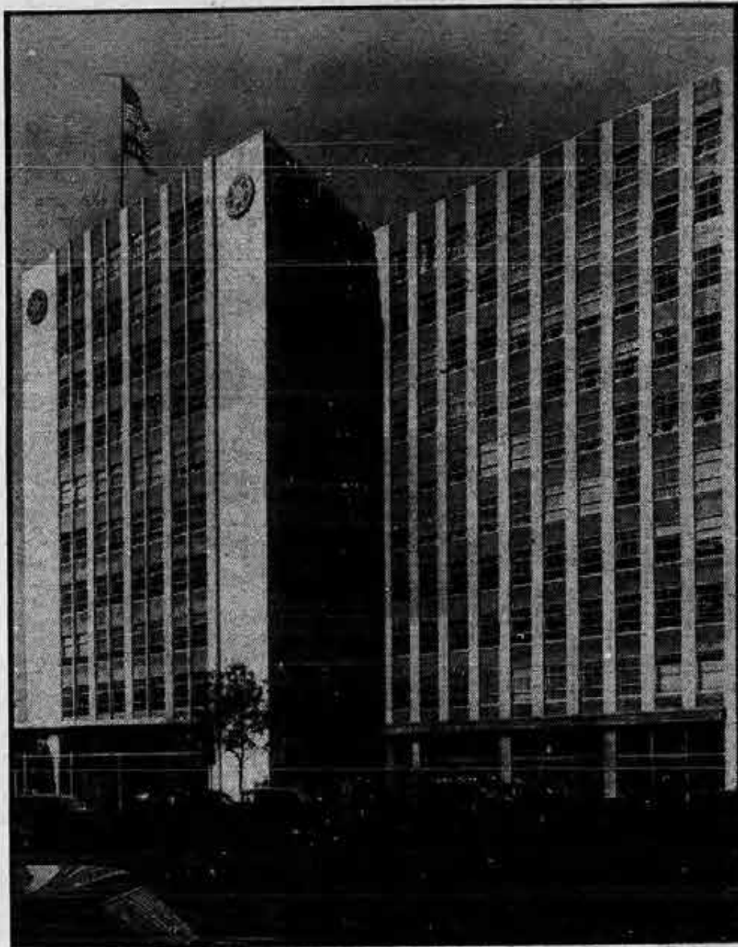
Impressive headquarters building in Washington is ten stories of reinforced concrete faced with marble. Union occupies about 60 percent of space, rents out rest.
