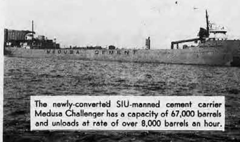
The newly-converted SIU-manned cement carrier Medusa Challenger has a capacity of 67,000 barrels and unloads at rate of over 8,000 barrels an hour.
