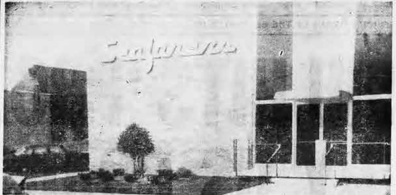
New "Seafarers" sign on exterior of the recently-opened SIU hall in Norfolk adds final touch to the one-story building. The modern structure, built so that an additional floor can be added later if necessary, opened for shipping and other business last November.
