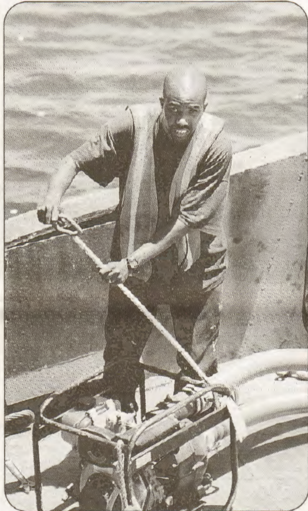
Engineer Apprentice Manuel Little works to repair a portable pump on board the tug Pioneer .
