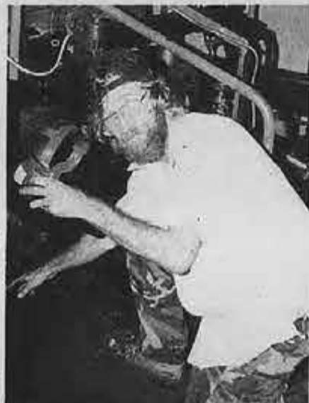
Checking on boiler operations is OMU Charlie Perryman.
