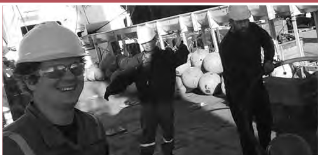
AB/Third Mate Tyler Brenton (left), AB/SJ Arsenio Brecio (center) and AB Paul Nelson apply floats to the umbilical cord of the Plough prior to launching it to begin the cable burial.
