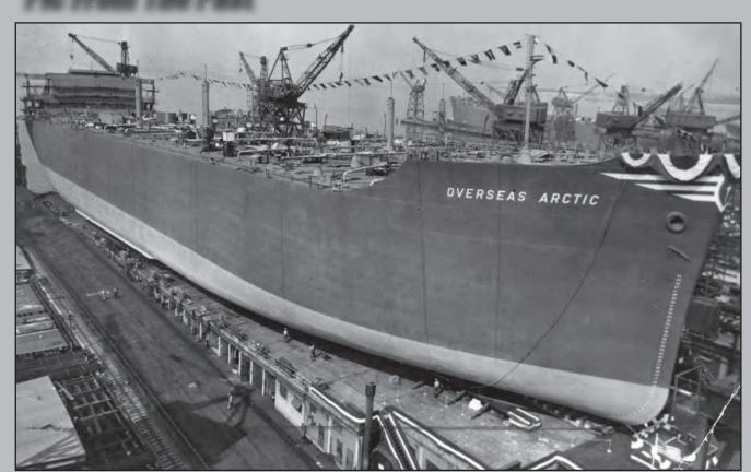
The SIU-contracted Overseas Arctic is pictured shortly before its launch in 1970. Built at Bethlehem Steel's Sparrows Point yard, the tanker weighed 62,000 dwt and had a capacity of 524,000 barrels. It could sail at 15.5 knots and was 731 feet long, with a breadth of 105 feet.
