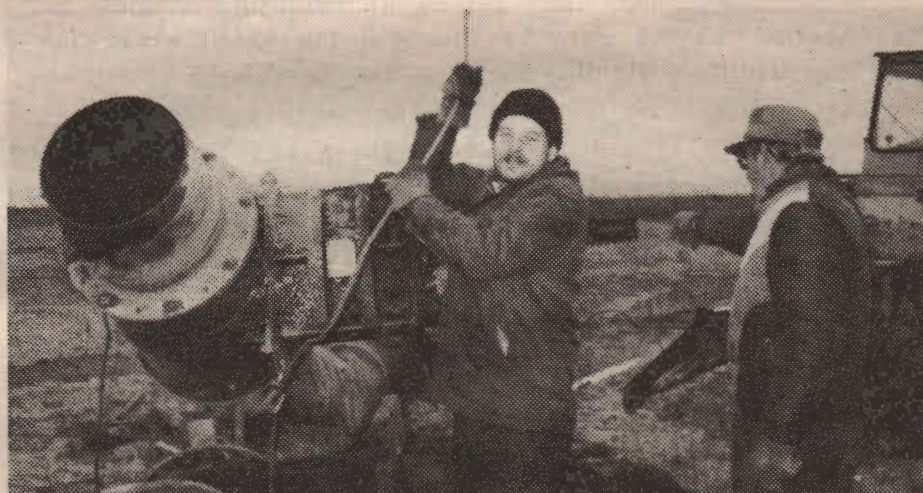
Seafarers Michael Lock (l.) and Bruce Lancaster prepare to add a "Y" valve pipe section to the landside dump area at Point Mouillee, Mich.
