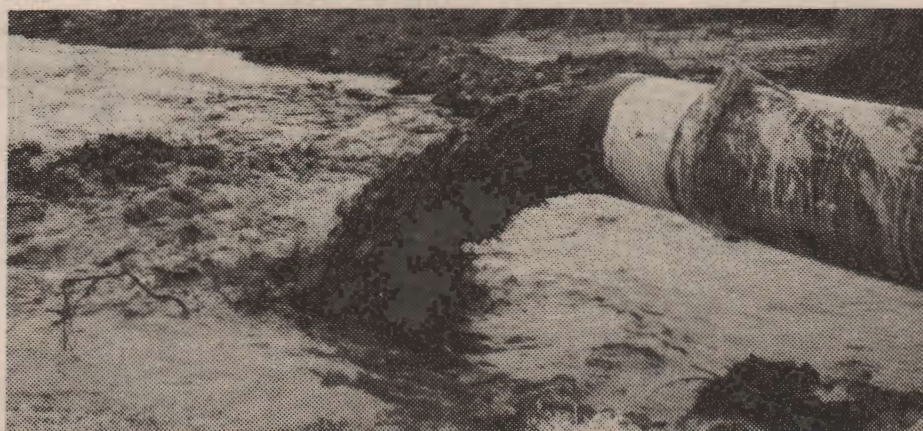
It's mud to most folks, but it's "black gold" to SIU dredgemen and tugmen who man the Dunbar & Sullivan equipment at Point Mouillee, Mich. The 36" pipe spews dredged material which has been loaded into scows and then sucked out by a hydraulic dredge and deposited 3,000 feet inside a diked disposal area.
